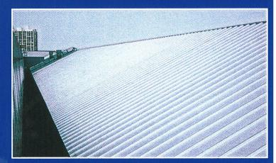
Ford chose a MR-24® standing seam metal retrofit roof system by Butler. The new MR-24 retrofit system utilized z-shaped subpurlins for attachment to the existing roof tiles. A layer of 4" fiberglass insulation was installed under the new roof panels providing significant long-term energy savings.
