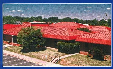
A VSR<sup>TM</sup> architectural standing seam roof and slope build up system by Butler was used to add pitch and enhance the appearance. Energy savings resulted from the addition of new insulation. The project was completed while the clinic remained completely operational.
