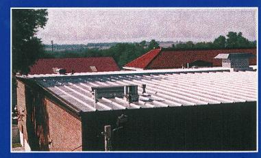
The gymnasium was reroofed with a complete Butler retrofit system that includes a MR-24® standing seam metal roof system installed on a structural slope build up system that added pitch to the existing flat roof. To lower the schools ongoing energy costs, a total of 9" of blanket insulation was added.
