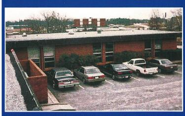
The Anderson Mental Health Center's roof was beyond repair. Three interconnecting buildings were plagued with so many leaks that patching wasn't even a consideration. The roofing felts and flashings contained asbestos, compounding the problem
