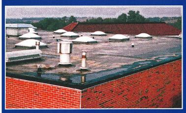
After numerous patch jobs and significant maintenance, this single-ply rubber roof installed over a school gymnasium failed in less than 10 years. Much of the insulation became saturated with water and had lost its effectiveness.
