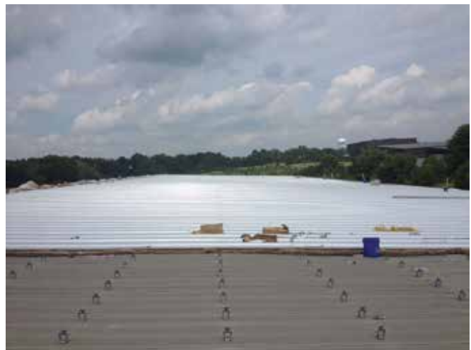
112,000 square foot Butler Re-Roof
