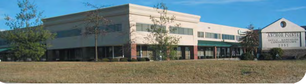
Lichtefeld provided construction services for the Anderson Monsour project in Louisville.
